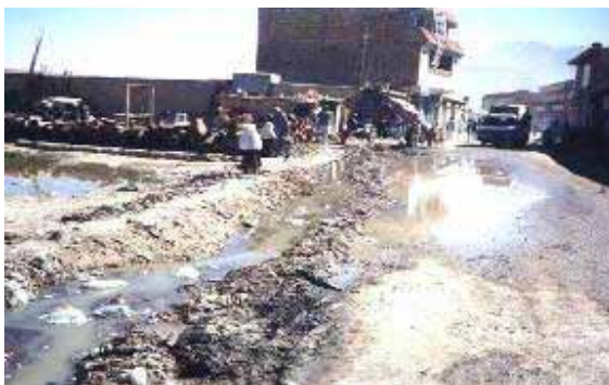
Prevailing situation in Katchi Abadies with sewerage water overflowing prior to intervention of QKAEMP
