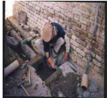
Mason constructing a manhole outside a house
